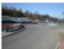
Most na Poddębice (Fot. 12)
