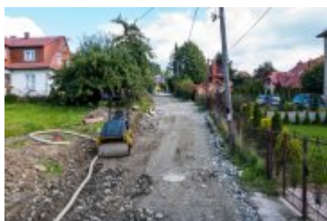
• 2021-09-03-Remont ulicy Tetmajera
