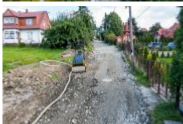
• 2021-09-03-Remont ulicy Tetmajera
