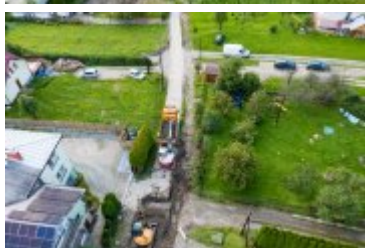
• 2021-09-03-Remont ulicy Tetmajera
