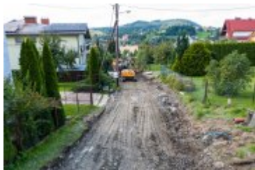
• 2021-09-03-Remont ulicy Tetmajera
