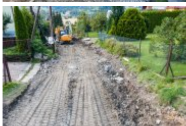
• 2021-09-03-Remont ulicy Tetmajera
