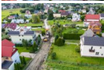
• 2021-09-03-Remont ulicy Tetmajera
