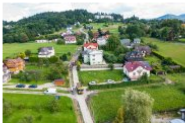
2021-09-03-Remont ulicy Tetmajera
