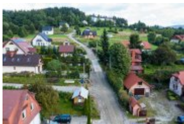
• 2021-09-03-Remont ulicy Tetmajera
