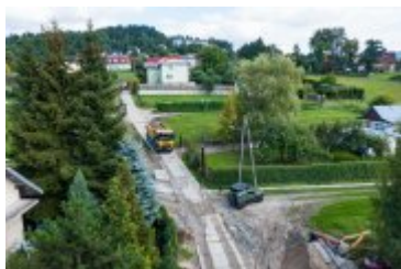
2021-09-03-Remont ulicy Tetmajera
