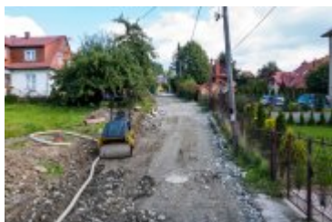
• 2021-09-03-Remont ulicy Tetmajera
