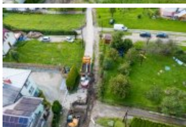
• 2021-09-03-Remont ulicy Tetmajera
