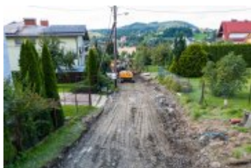
• 2021-09-03-Remont ulicy Tetmajera
