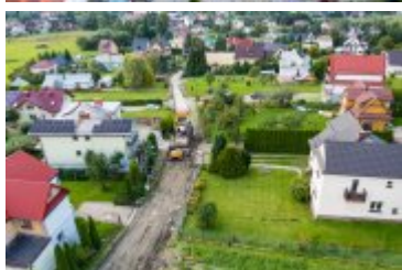
• 2021-09-03-Remont ulicy Tetmajera
