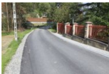
2021-09-07-Ulica Garncarska po remoncie
