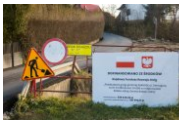
2021-11-07- Remont ulicy Tetmajera
