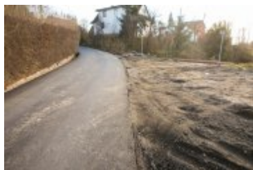
2021-11-07- Remont ulicy Tetmajera
